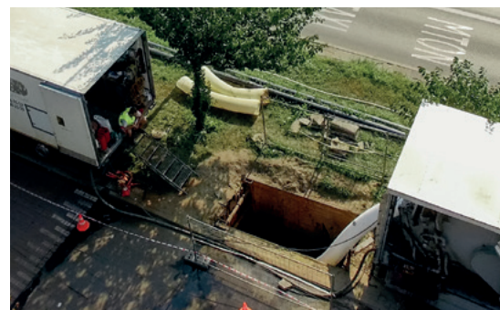
Liner installation with inversion system
