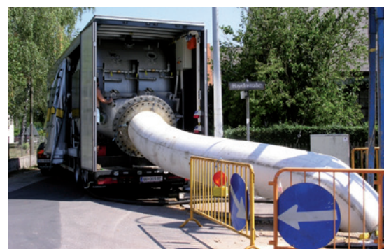
CIPP installation unit
