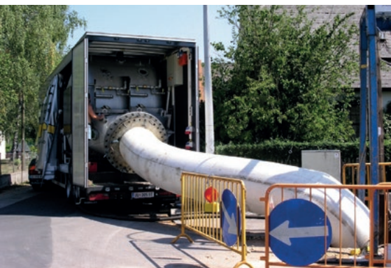
CIPP installation unit
